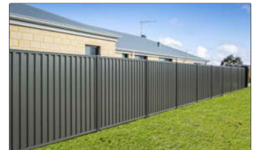
COLORBOND FENCE: 1.8mH PRE-COATED METAL SHEETING PANELS (STRATCO SUPERDEK) IN 'GREY RIDGE' COLOUR
